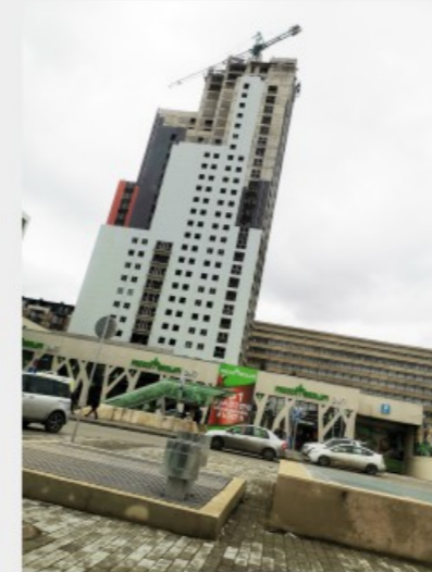
▲ Location: Georgia Project Name: SABURTALO PALACE
