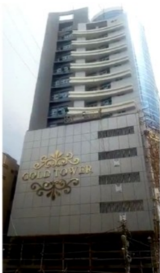
Location: Pakistan Project Name: Gold Tower
