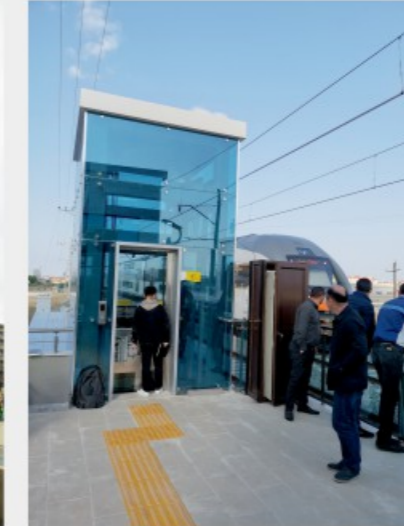
▲ Location: Azerbaijan Project Name: Railway station 24-1
