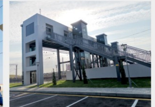
▲ Location: Azerbaijan Project Name: Railway station 24-21
