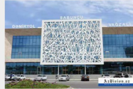
▲ Location: Azerbaijan Project Name: Railway station 24-15
